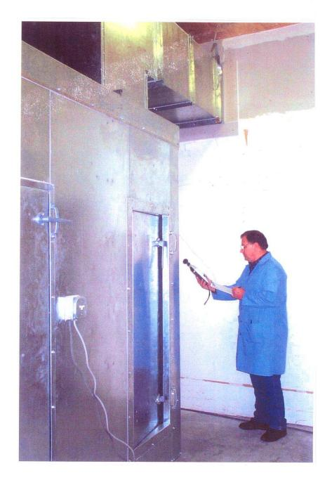
AIR ZONE publishes a casing leakage design of 1% or less at 10.0" W.G. and panel deflection not to exceed 1/250 of an inch.
